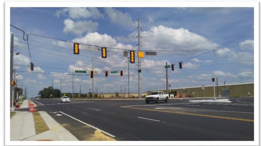
Figure 2 A new intersection improvement at US 84 East and Clay Road/Hollywood Street
