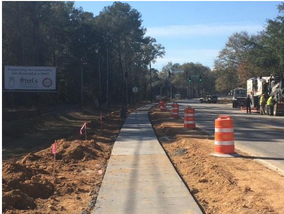
Figure 1 New sidewalk along Park Avenue, a federal aid Safe Routes to School Project near J.L. Newbern Middle School in Valdosta, 2015
