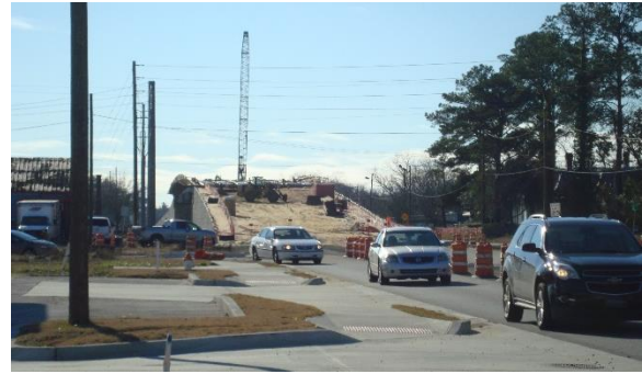
Figure 2 US 84 Overpass under construction near downtown Valdosta, project completed 2014.
