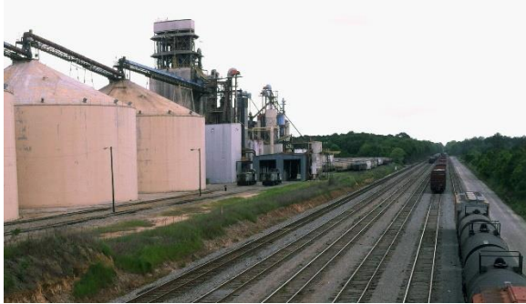
Figure 41 Norfolk Southern Railroad at Clay Road in Valdosta
