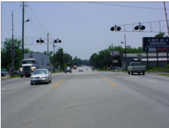
Photo WH-C3—Looking west along Hill Avenue just beyond the railroad tracks and potential overpass area.
