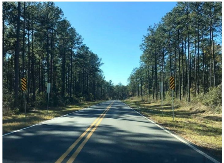
Pictured here is the newly constructed Arglass Road.
