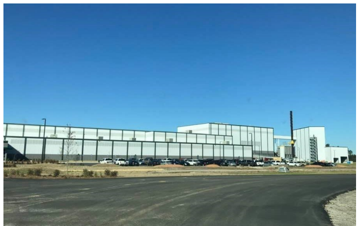
Arglass Yamamura glass manufacturing facility.
