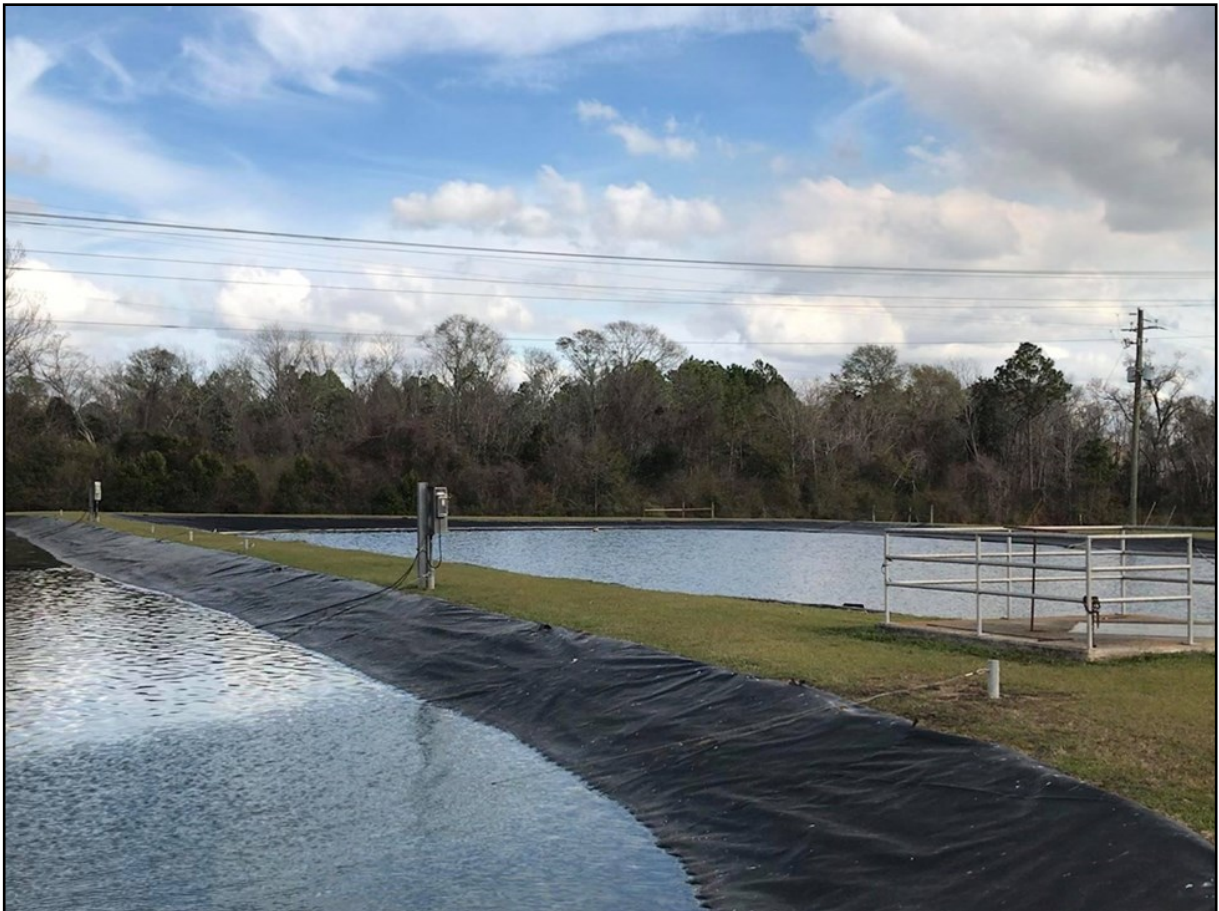
City of Sycamore Wastewater Treatment Facility
