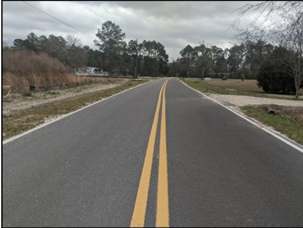
Street, Flood, and Drainage Improvements
