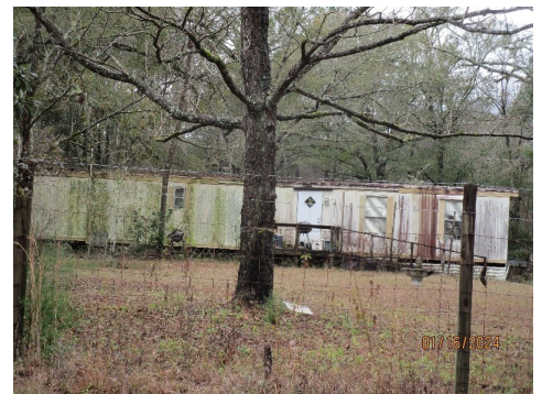
Right: A home within the Homeland Target Area in need of replacement.
