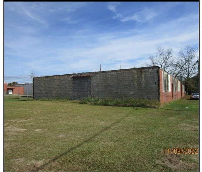
Demolition of existing building and construction of new recreation complex in Ben Hill County
