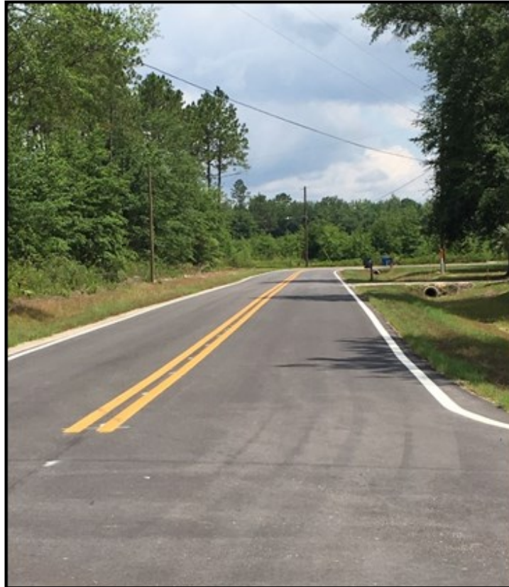
Street, Flood, and Drainage Improvements
