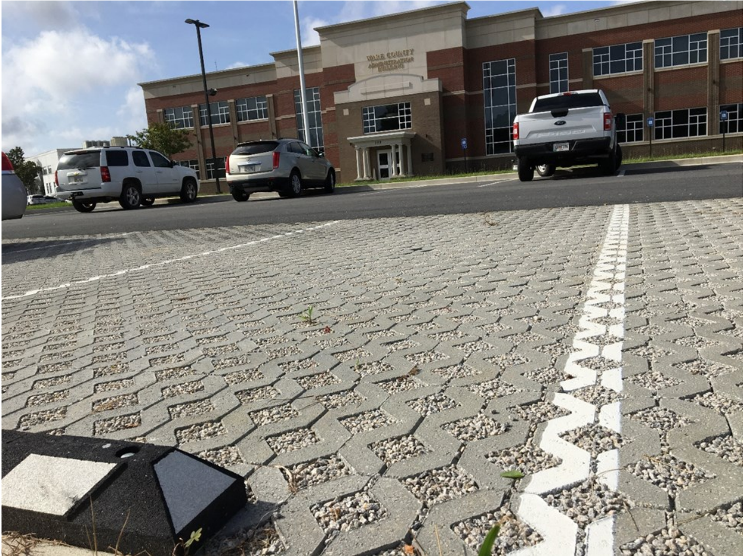
Pictured above: permeable parking lot at the new Ware County Administration Building.
