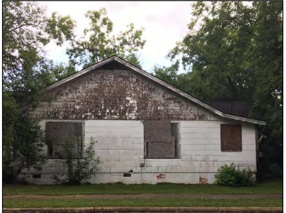
Pictured above is a structure surveyed in the city of Douglas
