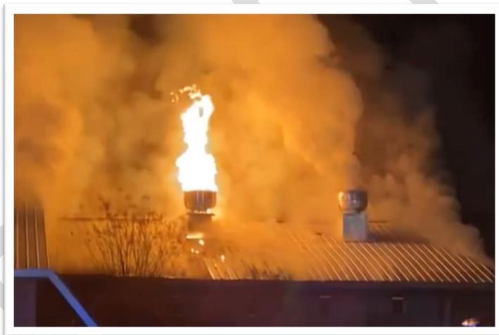
Country Cabin Restaurant Fire December 14, 2021
