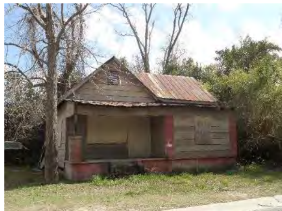
Figure 6: 920 I Street (Evans Way)
