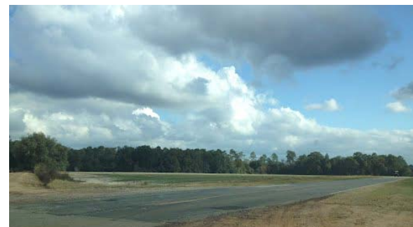
Figure 7 Typical roadway conditions in Cook County along Bike Route 15
