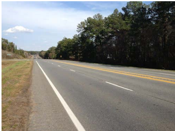
Figure 9 Bicycle Route 15 along Hwy 319, notice the rumble strips on the shoulder
