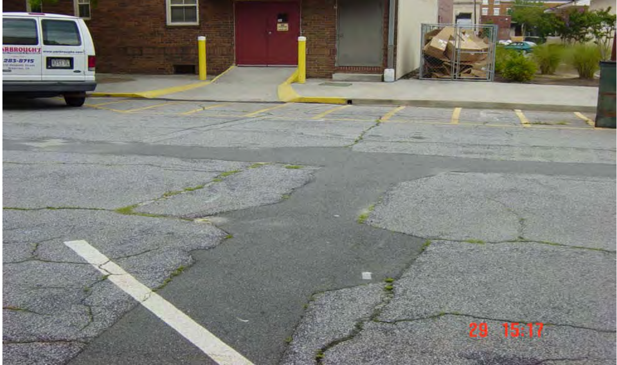
Loading Dock Incursion On West Side Of Parker Street Between Mary Street & Elizabeth Street
