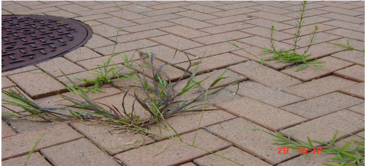
Broken Brick Island On West Side Of Parker Street Between Elizabeth Street & Jane Street
