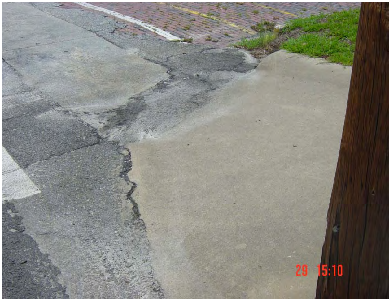
Bad Gutter To Pavement Heights At NW Corner Of Tebeau Street & Jane Street
