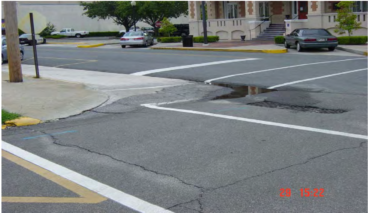
Reported Crossing Hazard At SE Corner Of Pendleton Street & Isabella Street
