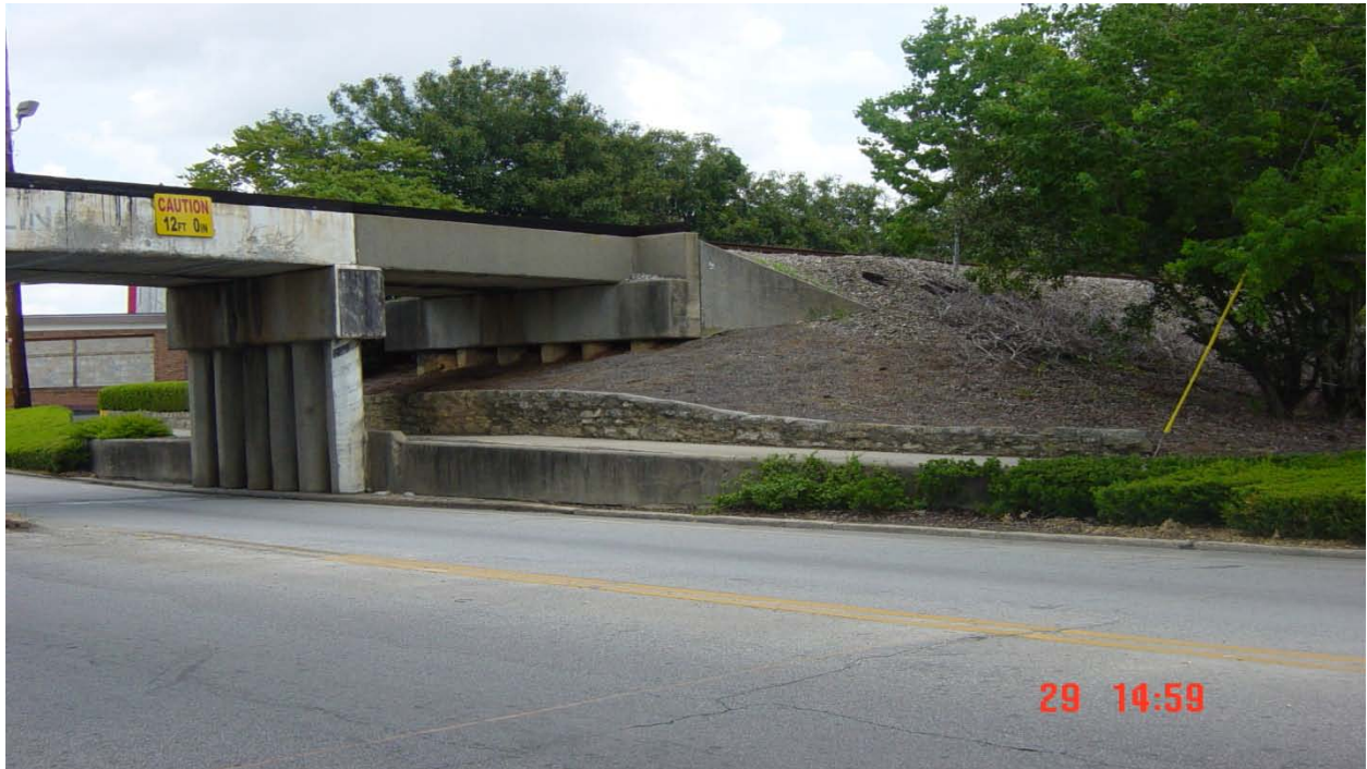
East Side Of Lee Avenue Between Knight Avenue & Memorial Drive
