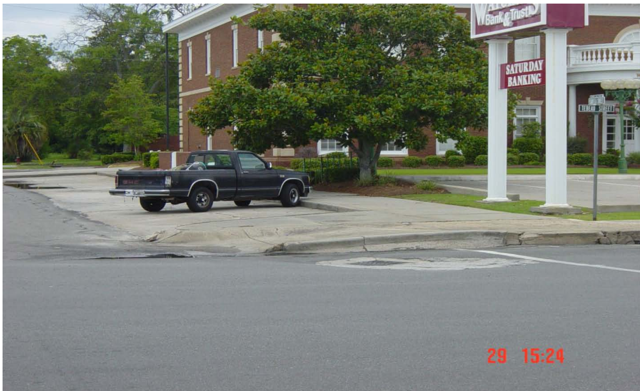
Dangerous Intersection At NW Corner Of Tebeau Street & Isabella Street
