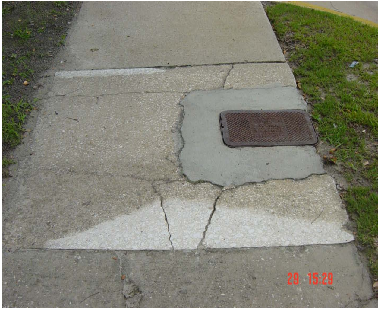
Ground Down Sidewalk Repair On SW Corner Of Carswell Avenue & Lott Street
