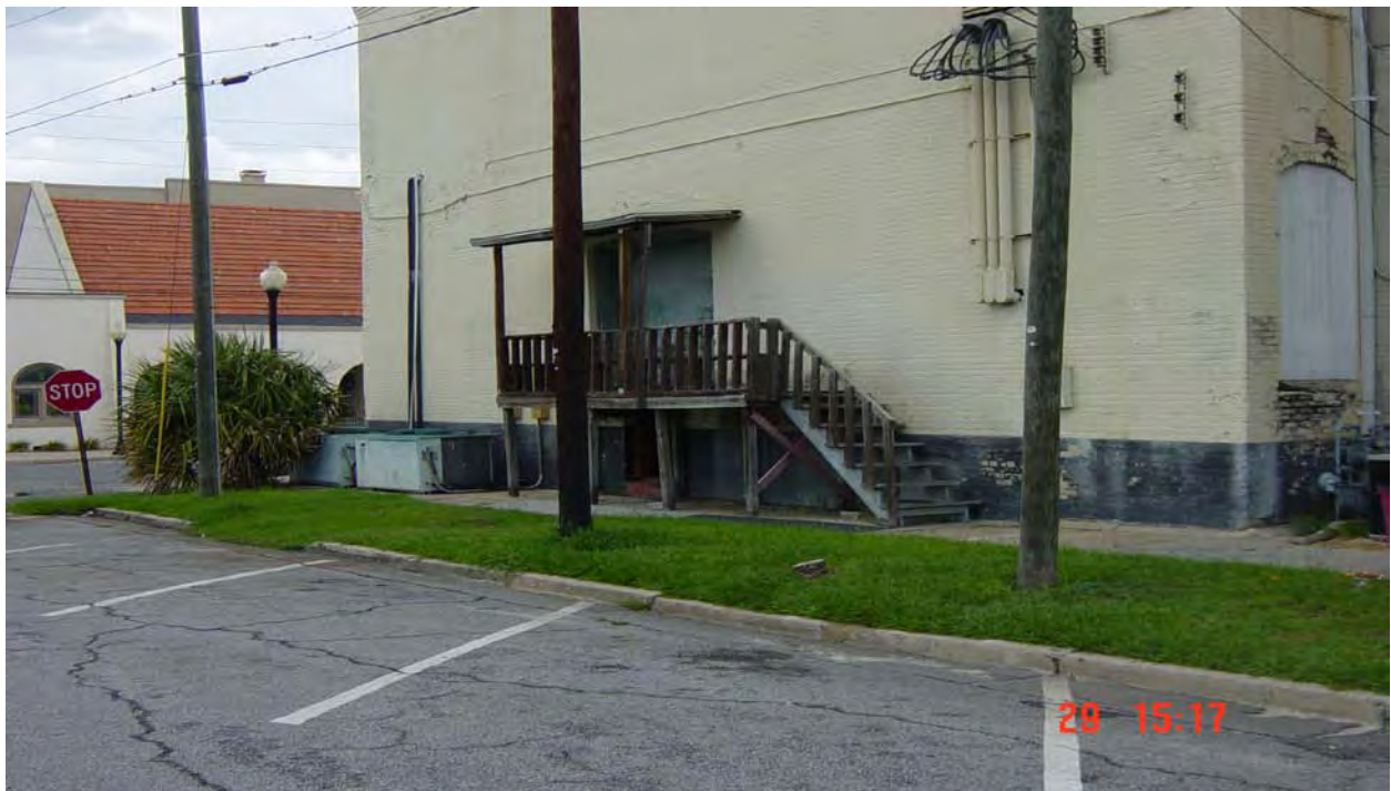
Porch & Air Conditioner Incursion On East Side of Parker Street Between Mary Street & Elizabeth Street
