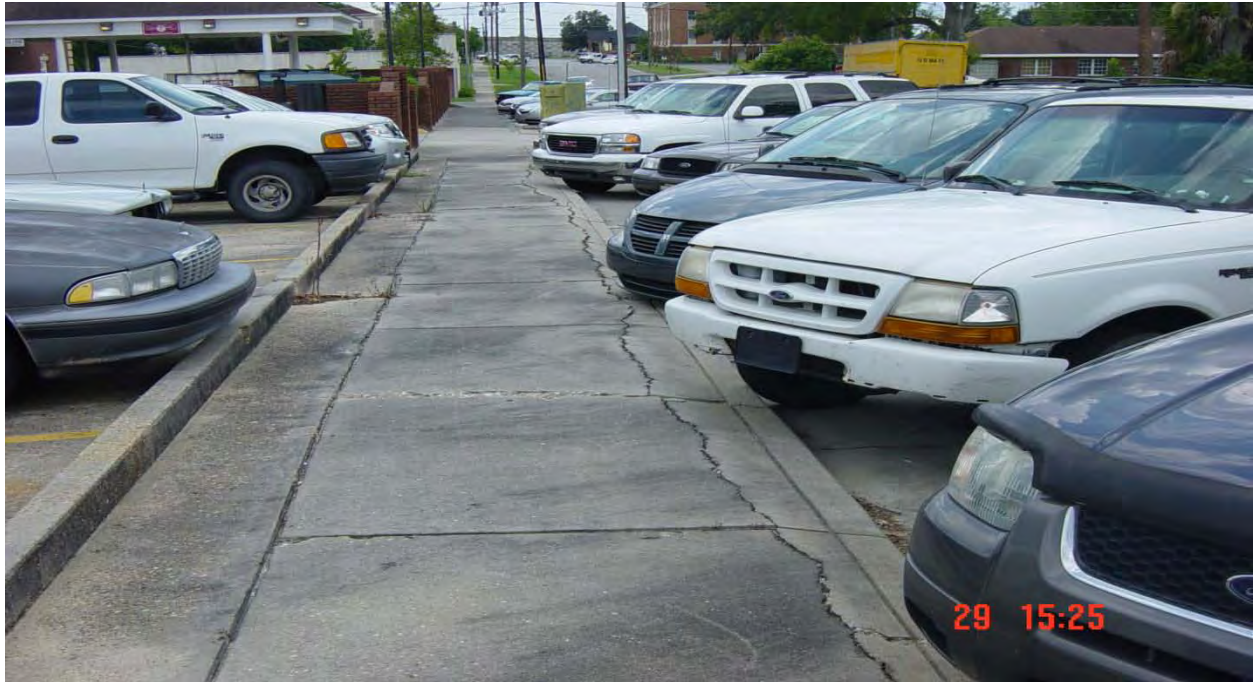
Curb Pulling Away From Sidewalk On East Side Of Remshart Street Between Carswell Avenue & Isabella Street
