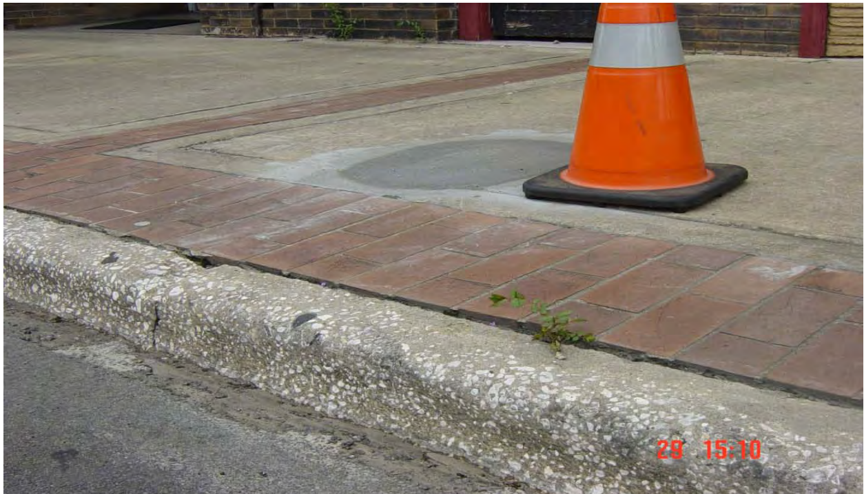
Curb Pulling Away From Sidewalk On East Side Of Remshart Street Between Carswell Avenue & Isabella Street
