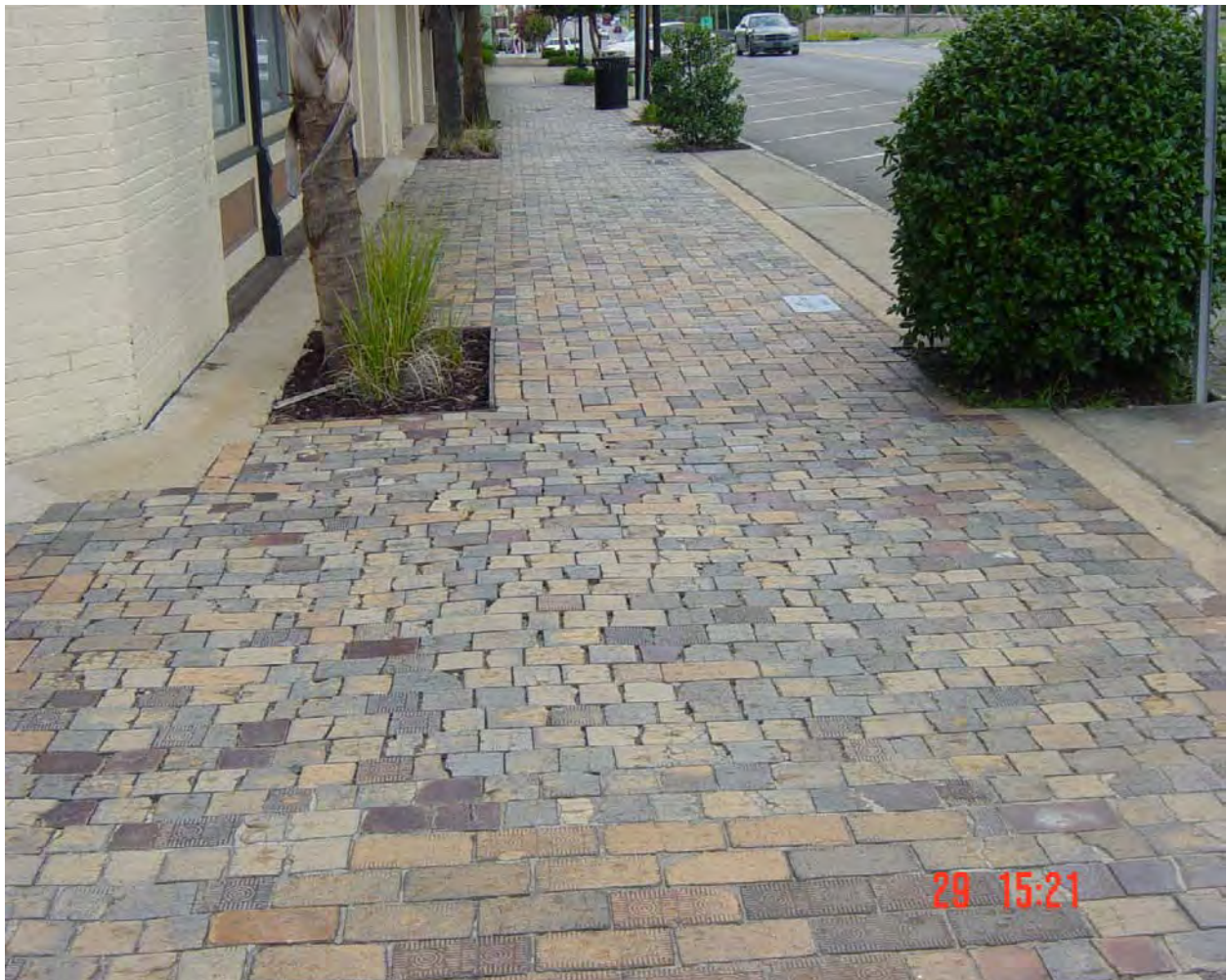
Broken Bricks-West Side Plant Avenue Between Isabella Street & Mary Street
