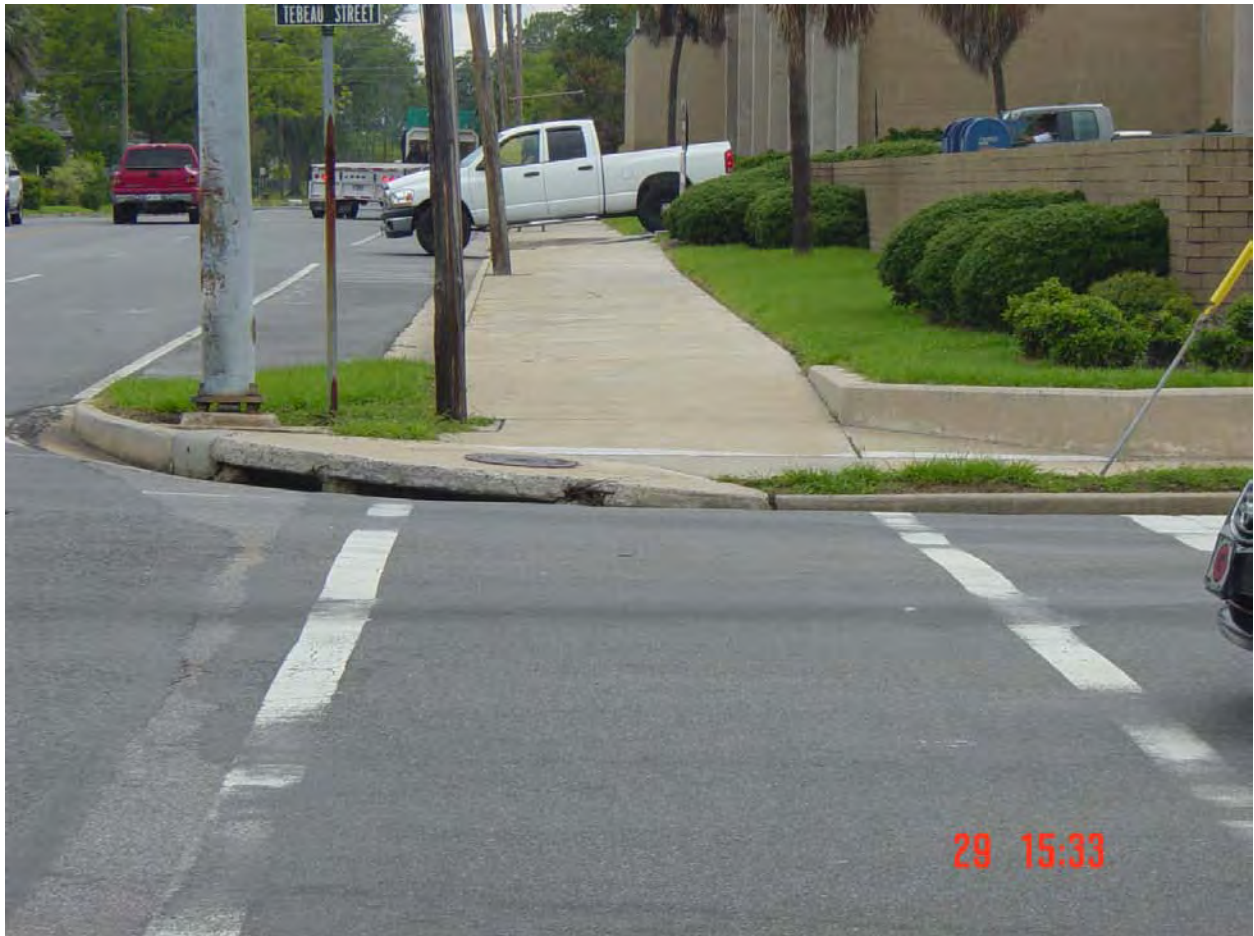
Drain At NW Corner of Tebeau Street & Carswell Avenue
