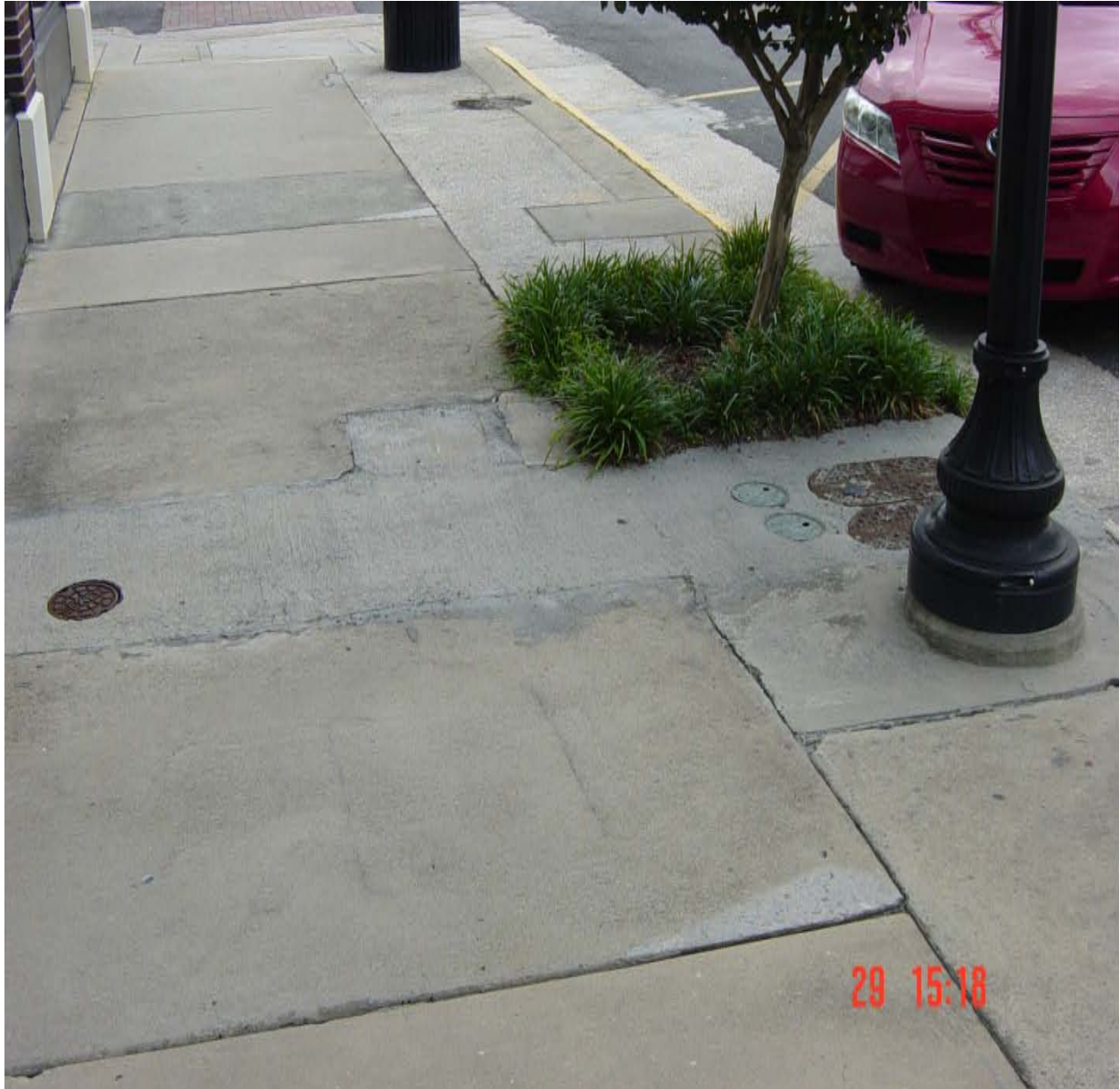
Bad Utility Cut On North Side Of Elizabeth Street Between Parker Street & Pendleton Street
