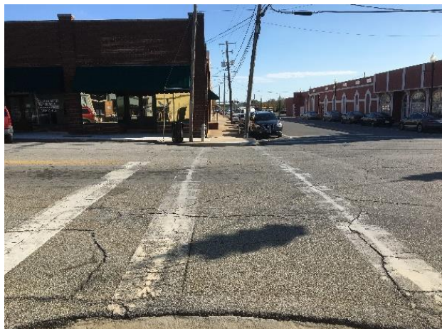
Figure 9. Deteriorated intersection crosswalk lacking perpendicular bars, Commerce Way.
