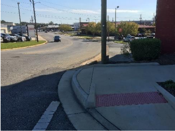
Figure 6. North view of sidewalk gap, Tift Avenue south of Third Street.
