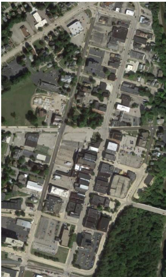
Figure 28. Aerial view of a community of comparable size (Ashtabula, Ohio) with a greater proportion of surface parking in the Downtown area, creating a less inviting environment.
