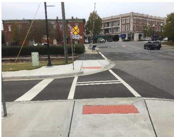
Figure 3. Parking lot exit with crosswalk and ADA ramps on Main St.
