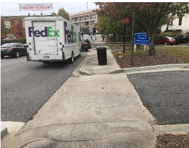
Figure 2. Parking lot entrance without crosswalk, and blocked sidewalk on Main St.
