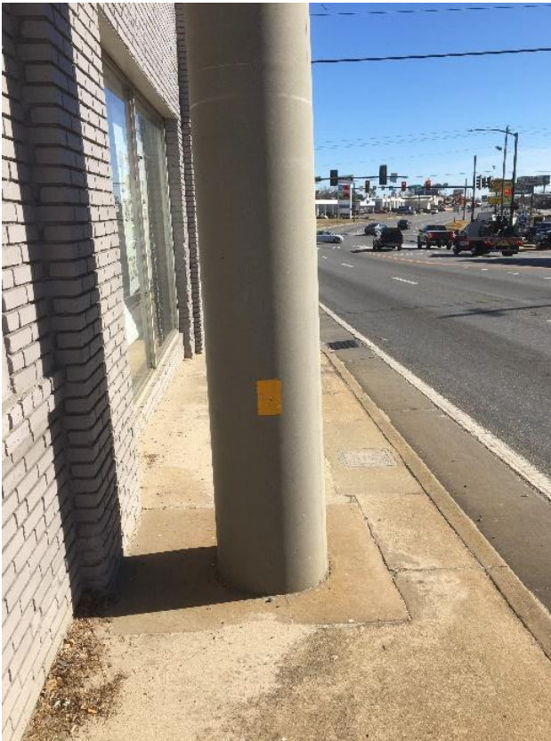
Figure 12. Utility pole blocking sidewalk on Fifth Street.
