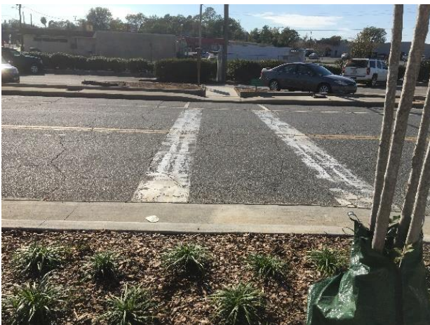
Figure 8. Deteriorated mid-block crosswalk lacking perpendicular bars, Commerce Way.
