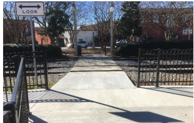
Figure 11. The smooth concrete pedestrian railroad crossing between Brumby Way and First Street is more inviting to pedestrians, and includes an advisory sign for safety.
