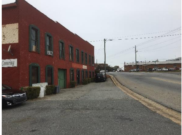
Figure 7. South view of sidewalk gap, Tift Avenue south of Third Street.
