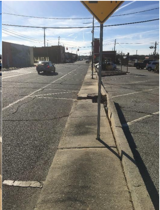
Figure 13. Obstructed and deteriorated sidewalk on Commerce Way.
