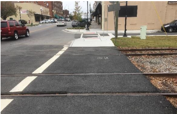
Figure 10. Asphalt sidewalk railroad crossings are less inviting to pedestrians, and can be difficult for wheelchair and stroller users to negotiate.
