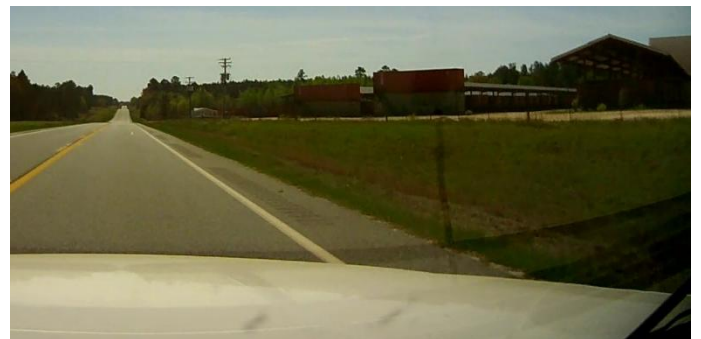
Figure 16 Wider Shoulders along Hwy 206, north of Douglas, GA
