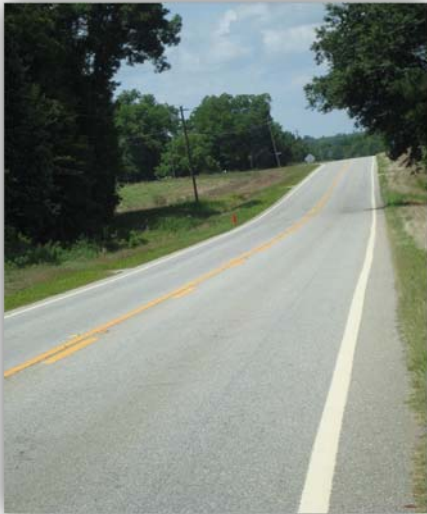
Figure 19 Typical Rural Highway, Highway 76 in Brooks County
