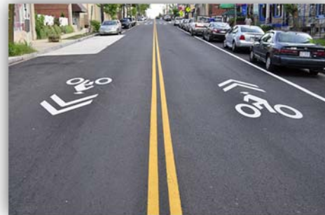
Figure 11 Typical Downtown Sharrow Application
