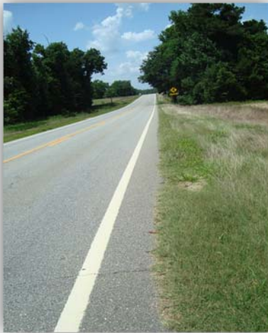
Figure 7 Typical Rural Highway, Highway 76 in Brooks County
