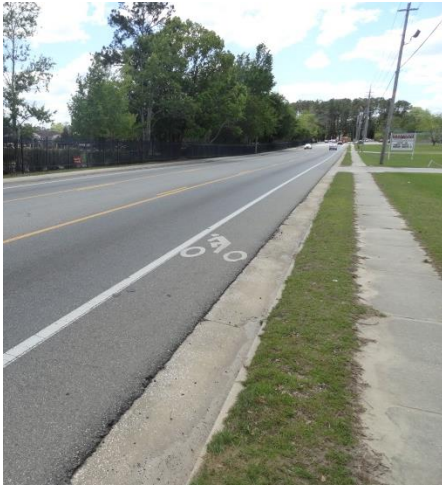
Figure 5: Bike lane on Lankford Drive
