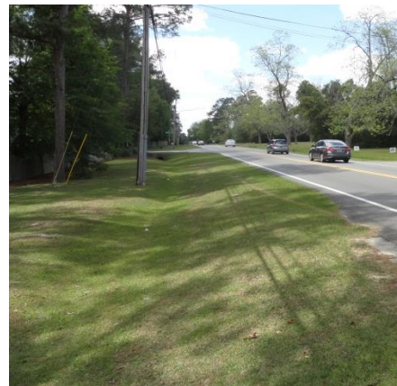
Figure 6: Stormwater ditches, like along Eager Road, are not conducive to immediate Complete Street projects
