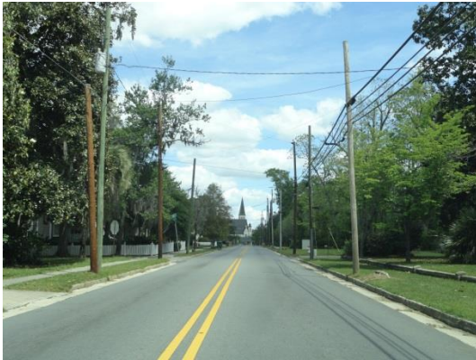
Figure 7: Utility poles on the ROW along River Street
