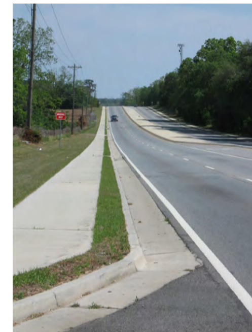
Bemiss Road - Bike Facilities Needed
