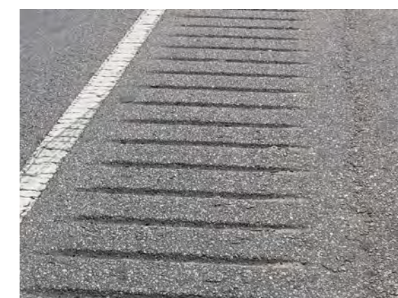
GDOT Rumble Strips - Old
