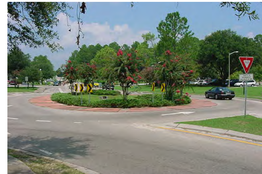
One-Lane Roundabout (Tallahassee, Florida)
