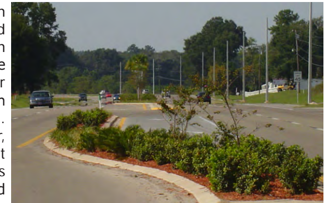
Turn Lanes with Landscaped Median
