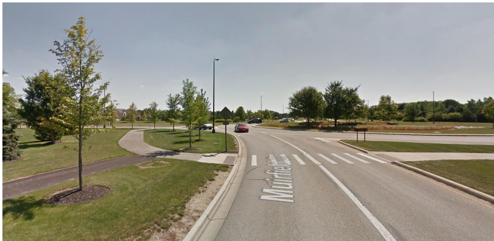
Figure 2. Example of a roundabout with marked crosswalks and connection to a multi-use trail. (Dublin, Ohio; Source: Google Street View)
