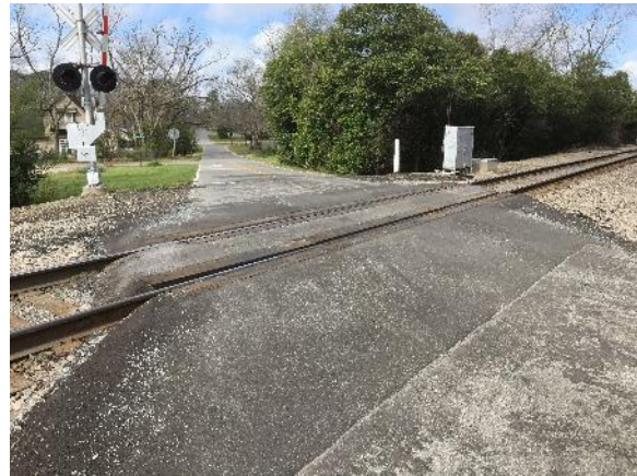
Figure 9. Angled railroad crossing on West Oconee Street.
