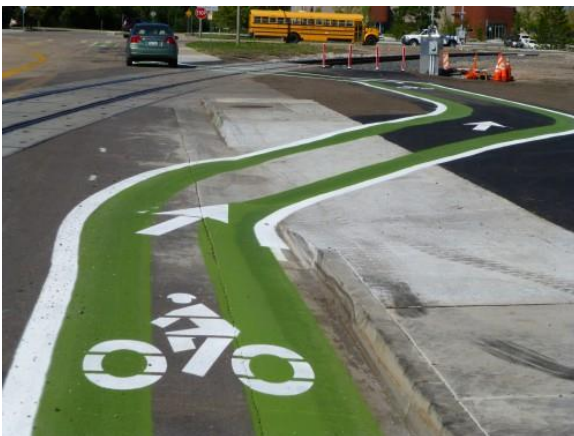
Figure 11. Example of a bike lane that is angled to guide bicyclists to cross railroad tracks safely. Source: Adam Farabaugh, ILoveBicycling.com
