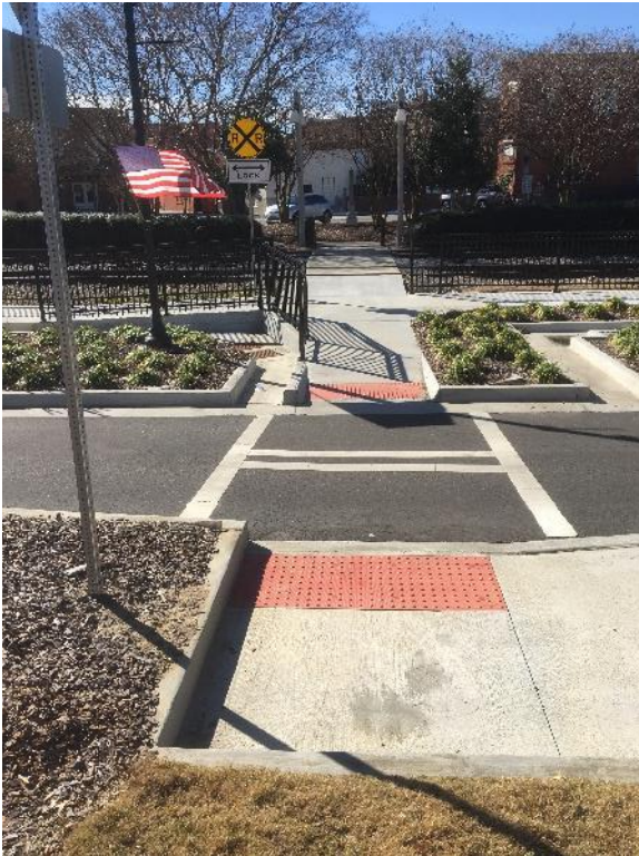
Figure 15. South-facing view of improved pedestrian railroad crossing in Tifton. (Photo: Ariel Godwin)
