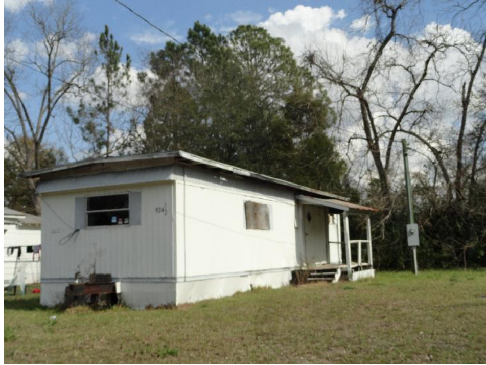
Figure 13: 924 1-2 Albert Hill Sr. Drive
