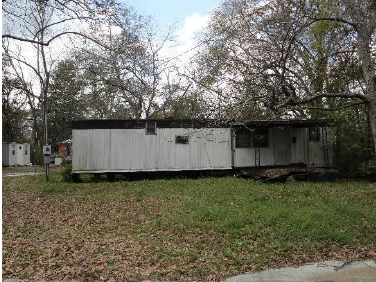
Figure 3: 805 Vernon Willis Drive
